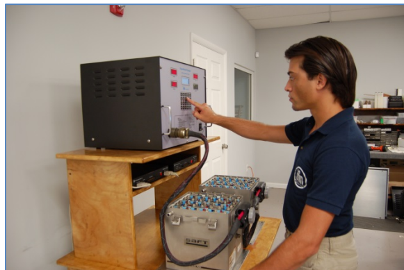
Figure 14 – Charger-Analyzer and Batteries placement
